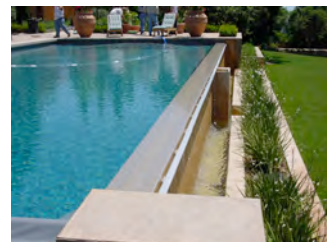
Topguide mounted using brackets on side of pool
