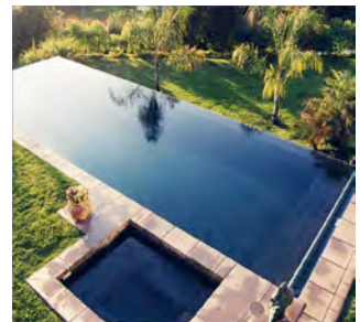
Double vanishing edge side and end of pool
