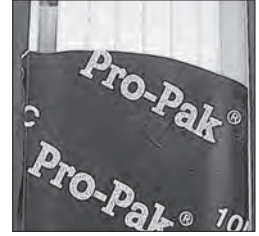
(3) Guide protected by 2" 10 mil plumbers tape
