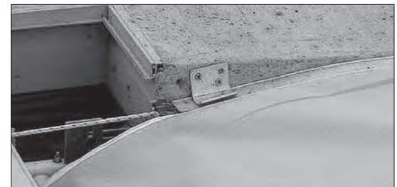
(6) OPTION: Recessed horizontal guide sloped into the box. Purchase set of curved guides for housing end of guide. Bend begins 15" in front of housing. Make sure top of guide is minimum of 1" lower than bottom of lid.
