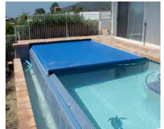
Vanishing edge using topguide on side of pool
