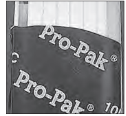
(3) Guide protected by 2" 10 mil plumbers tape
