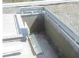
Box Perimeter Forming
