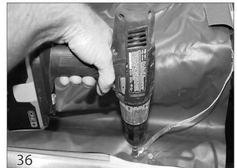
Lay the bond wire on top of the cover fabric. Secure it to the roll up tube using a tek screw (32).
