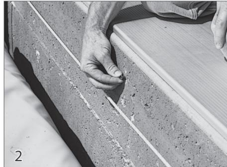
Insert plastic anchors in each of the holes that were drilled. Tap the anchors (33) with a hammer so they are in the hole completely.
