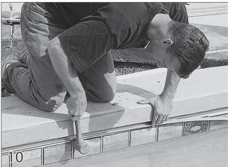
10 Insert and tap the spacer into place underneath the track along the entire length of the track. Do this along both sides of the pool. The spacer needs to end at the inside edge of the cover box.
