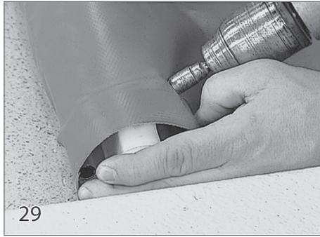
Position the fabric on the leading edge so it is in line with the leading edge support bracket. Secure with a 10 x 1/2" tek screw (31) on the back side of the leading edge tube. Be sure the screw does not interfere with the leading edge insert. Do this for both sides of the cover.
