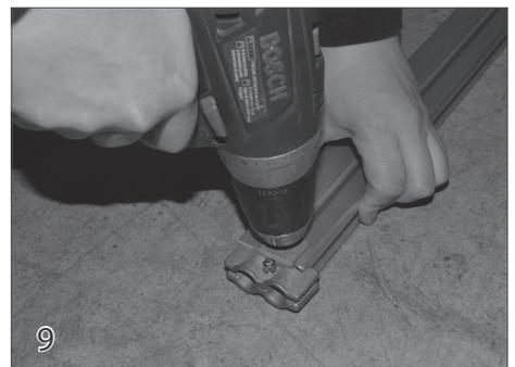
While holding the guide feed firmly, use a drill with a 3/16" bit to drill through the hole in the guide feed and through the track. Remove the guidefeed. Do this for the track on both sides of the pool.
