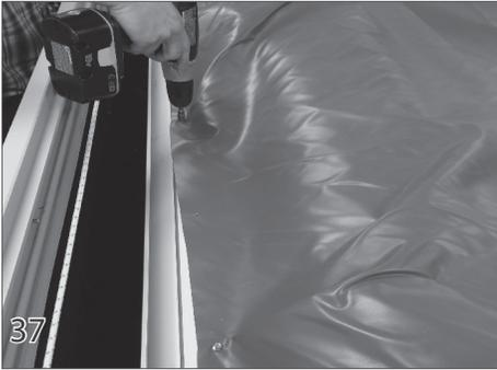
Distribute the slack of the cover evenly between each screw across the length of the tube. Secure the cover to the roll-up tube using tek screws (32) every 2-3ft.
