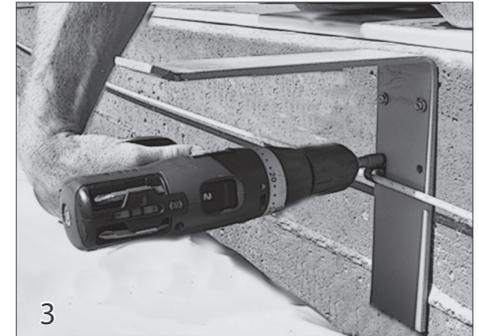
Secure the brackets to the back wall of the housing using #12 x 1 1/2" hex head screws (34). Mount a rope loop (30) on one screw of each of the brackets. This will keep the rope running straight along the back of the housing.
