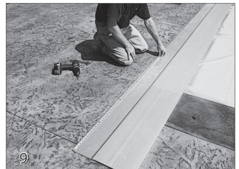
Measure across the hinge to evenly space the screws. Continue drilling and anchoring the hinge in this manner until the entire lid is attached to the deck. The safety pool cover installation is now complete. Now instruct the home owner using the home owners guide and the checklist on the next page.
