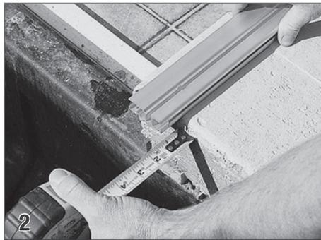
Cut the guide so it will extend from the front edge of the coping at the far end of the pool to 1" past the inside of the housing if no encapsulation is being used. When encapsulation is used, it will extend one inch past the inside of the housing, with the guide extending one inch past the end of the encapsulation.
