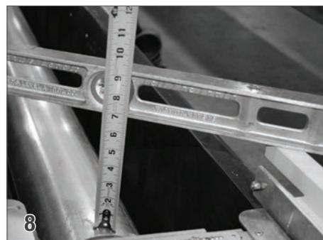
With the mechanism and tube assembled and set in place in the housing, check the roll-up tube for level. **This is crucial to proper operation of the cover.**
