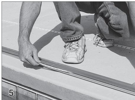
Hold the rope outside the guide to pull the rope down the length of the guide toward the end of the pool.
