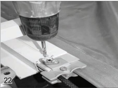
Drill through the center of the encapsulation and guide. Insert a 10-32 x 1 3/4" screw (42) and nylock nut (29). This step is very important. This will prevent the guide from sliding into the cover housing during the operation of the cover system.
