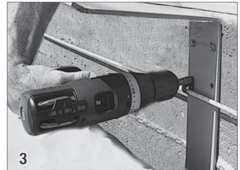
Secure the brackets to the back wall of the housing using #12 x 1 1/2" "hex head (34) screws. Mount a rope loop (30) on one screw of each of the brackets. This will keep the rope running straight along the back of the housing.
