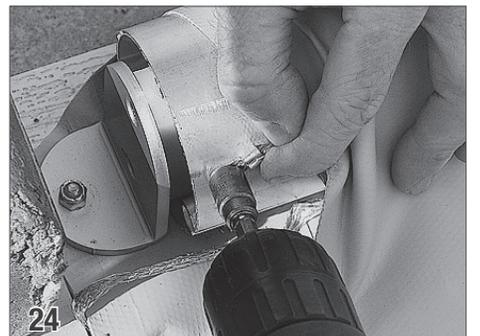
Connect the bonding wire that is attached to the front corner of the cover to the leading edge bar using a tek screw (32). Be sure the screw doesn't interfere with the leading edge insert.
