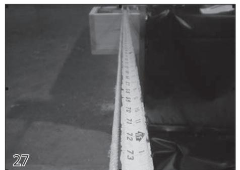
Leaving an extra 6-8 feet of extra rope length, pull on the ropes until the leading edge begins to move forward equally on both sides. Burn or wrap the rope with tape and cut to length.
