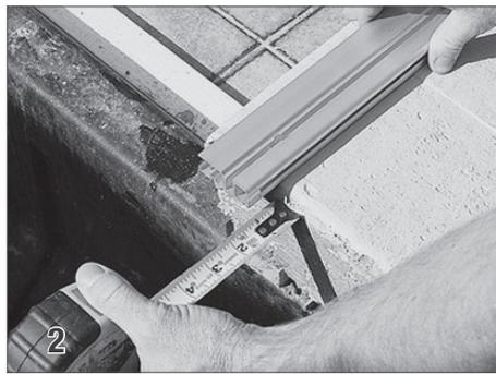
Cut the guide (14) so it will extend from the front edge of the coping at the far end of the pool to 1" past the inside of the housing if no encapsulation is being used. When encapsulation is used, it will extend one inch past the inside of the housing, with the guide extending one inch past the end of the encapsulation.
