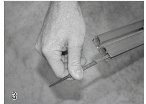
Before splicing the sections of guide together, file all guide ends thoroughly, rounding all edges and removing all burrs. **This step is extremely important!**
