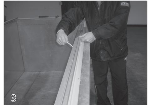
Pull the rope along the water side of the track towards the pulley end cap. Tip: Sometimes a guide feed can be put on to help feed the rope.
