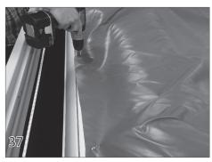
Distribute the slack of the cover evenly between each screw across the length of the tube. Secure the cover to the roll-up tube using tek screws (28) every 2-3 ft.
