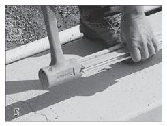
Lay the sections of track on the deck and tap them together using a rubber mallet so the center splice and splice pins interlock with each section of track.
