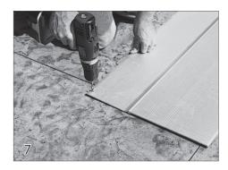
Attaching the Lid to the Deck Drill through the lid hinge along the back edge every 2'-3' using a 1/4" drill bit. Then, drill through these holes and into the concrete deck using a 1/4" masonry bit.
