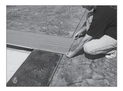
Position the lid over the top of the housing. The motor end and non-motor ends should extend past the cover housing 1-2". If they extend more and do not lay flat on the deck, it may be necessary to cut the lids. Mark the lid with a square at the 1" overlap point and cut it to length with a hacksaw or power saw with carbide tipped blade.
