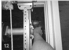
Anchoring the Mechanism Feet With the mechanism centered between the tracks and centered in the cover box front to back, anchor the mechanism mounting feet into the cover box. Use the appropriate screws and anchors depending on the type of cover box being used.
