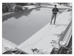
Attaching the Ropes to the Reels The cover must be open when cutting and attaching the ropes. Pull the cover back until the sliders are against the guide feeds. Pull the ropes tight as they come off the pulleys on the mechanism to eliminate the slack in the rope.
