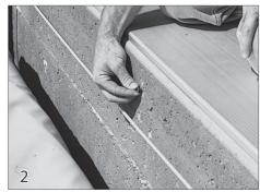
Insert plastic anchors in each of the holes that were drilled. Tap the anchors (29) with a hammer so they are in the hole completely.
