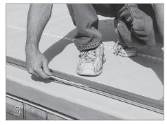
Hold the rope outside the track and pull the rope along the length of track toward the end of the pool.
