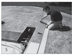
Slide the motor and non-motor lid ends onto the hinge.
