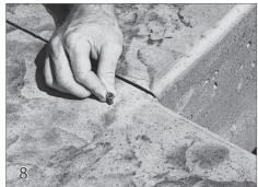
Insert plastic anchors (29) into the holes and tap with a hammer so they are flush with the deck. Fasten the lid to the deck with #12 pan head screws (23).
