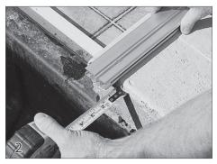
Cut the length of the track on each side of the pool so it will extend 1 inch past the end of the encapsulation into the cover box.
