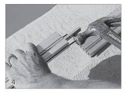
Tap the splice pins (33) into one end of the track and slide the center splice (21) into the center channel.
