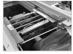
Positioning the Mechanism Lower the assembled mechanism with attached roll-up tube into the cover box and place it roughly in the position it will anchored. Note: If the cover box isn't square to the pool, position the mechanism in the cover box so it will be square to the cover track.
