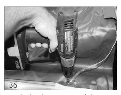
Lay the bond wire on top of the cover fabric. Secure it to the roll-up tube using a tek screw (28).
