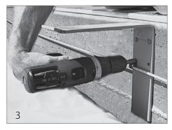
Secure the brackets to the back wall of the housing using #12 x 1-1/2" hex head screws (30). Mount a rope loop (27) on one screw of each of the brackets. This will keep the rope running straight along the back of the housing.
