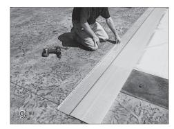
Measure across the hinge to evenly space the screws. Continue drilling and anchoring the hinge in this manner until the entire lid is attached to the deck. The pool cover installation is now complete.
