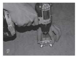
While holding the guide feed firmly, use a drill with a 3/16" bit to drill through the hole in the guide feed and through the track. Remove the guide feed. Do this for the track on both sides of the pool.
