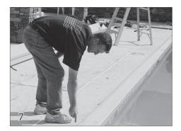
Pull the rope down the back side of the track toward the cover box.
