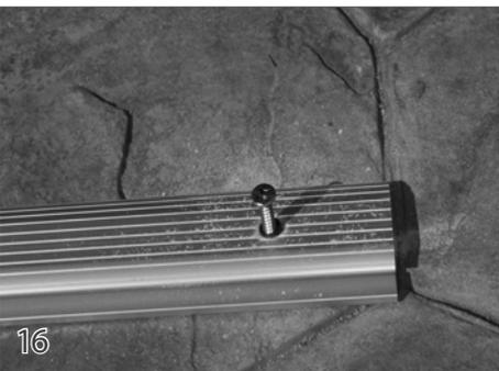
Place the track back over the holes in the deck. Fasten the track screws (15) halfway through the tracks into the plastic anchors. The screws will be fastened completely later in the installation.
