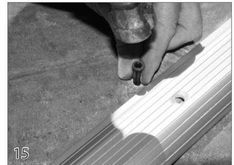
Move the tracks to the side to expose the holes in the deck. Tap the plastic anchors (25) into each hole.
