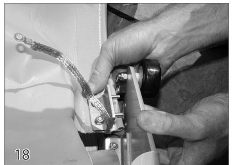
18 Connect the two hole bracket that is attached to the front corners of the cover to the wheel assemblies.
