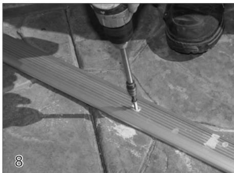
Complete the fastening of all track screws (17) and insert the pulley housing into the end of the track. Clean concrete dust from track and pulley end cap. Make sure ALL screws are flush with the top of the tracks.
